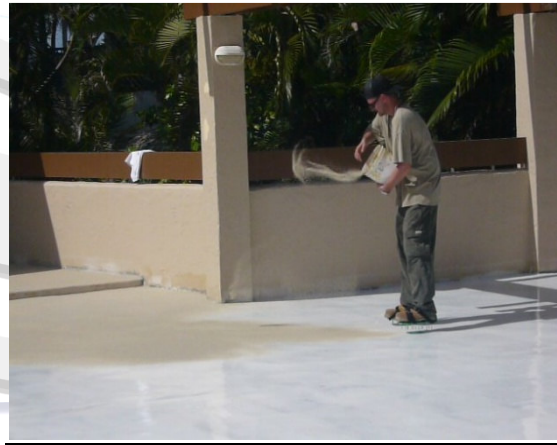
#14 Broadcast 16-40 mesh silica sand to refusal or until the deck looks like a beach.
