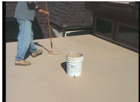
#16 Mix 3 qts of xylene into a five gallon pail of top coat. Apply evenly with a ½"-3/4" nap roller.
