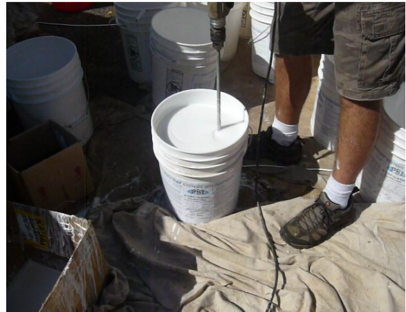
#6 Open can and mix the entire pail from the bottom to the top for 2 minutes.
