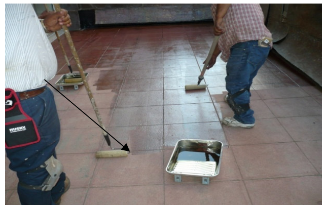
#4 IT IS NOT NECESSARY TO PRIME CLEAN PLYWOOD. Apply (to concrete) primer with 3/8" at a very thin rate of 300 sq/ft per gallon.
