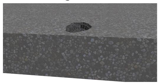
Layout and mark spall or void blockout 2" minimum to either/all sides of the desired repair area and a minimum of 2" deep.
