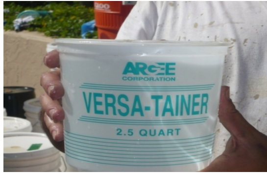
#6 Using a 2 ½ quart container, fill with water and pour into one of the 2 ½ gallon pails of coating .
