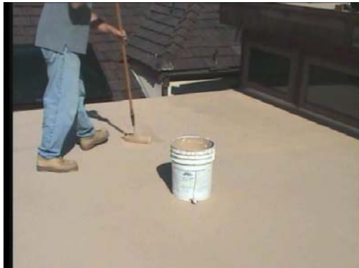
#14 Use a good quality 3/8" to 1/2" nap roller and apply Top Coat evenly without lap marks and puddles. Apply @ 80 sq/ft p/gallon.
