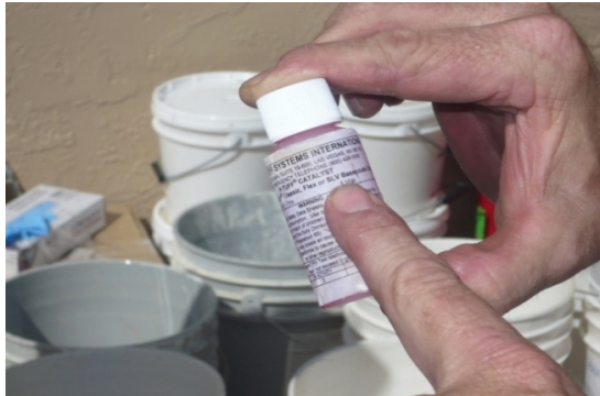
#7 Pour ½ vial of catalyst (green or pink) into the water before mixing. Use less or no catalyst in the heat, more catalyst in the cooler temperatures.
